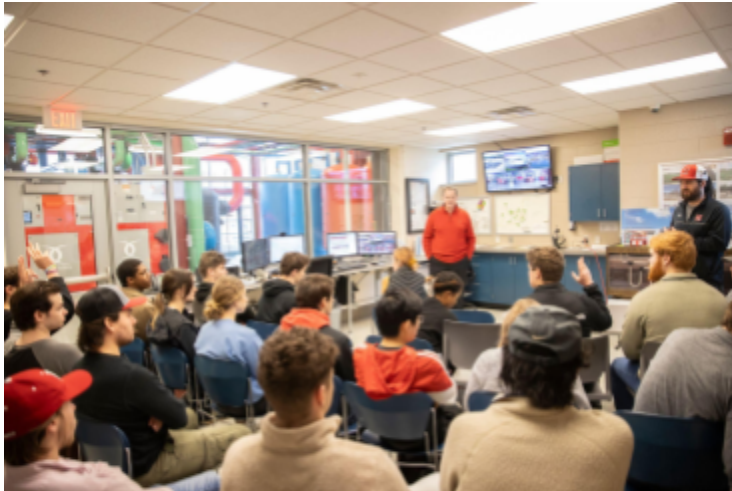
Larry Davidson, hydronics operations systems manager, talks to a group of students about geothermal exchange in the Western Geothermal Plant. Tours of the geothermal plant are offered to classes, student groups, community groups, and other visitors throughout the year.
