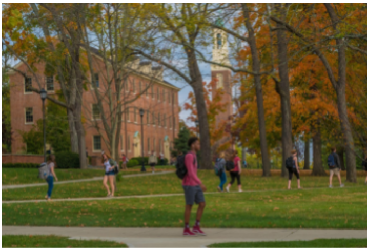
Elliott Hall, one of the oldest residence halls in the country, was one of Miami's first buildings converted to geothermal heating and cooling.
