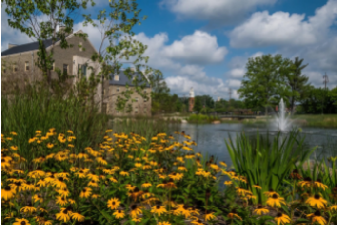
Approximately 300 geothermal wells are situated under Western Upper Pond (pictured above) and Lower Pond (a first-of-its kind use). Coils of piping, buried under the sand of Upper Pond, act as a heat exchanger and can provide the heat exchange of 30 geothermal wells.
